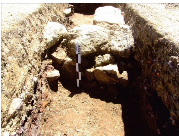
Fig. 32. 2 nd plan of the S1 trench, outlining the south-eastern wall; view from the exterior (photo by the authors).
